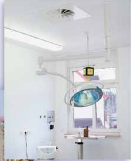
Giengen Dispanseri, Giengen / D Puridral ve Puri Inlet
