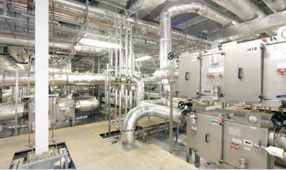
Several HEPA Filter housing with dampers installed and commissioned.
