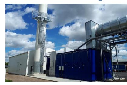
The use of a microturbine is very efficient in terms of energy if electricity and heat are needed at the same time as the VOC emissions are emitted during production. The heat demand should be as high as the heat output of the CHP unit throughout the year. Even large exhaust air volume flows can be co-combusted in a microturbine if a concentration unit for exhaust air treatment is installed upstream as the first stage.
