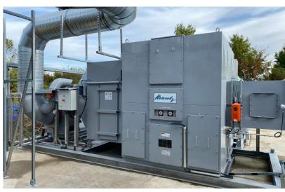
Due to the high VOC concentration in the desorbed air, the oxidiser is usually operated autothermally without additional fossil fuel consumption. Often, additional surplus heat can be used through the operation of an external heat exchanger.
