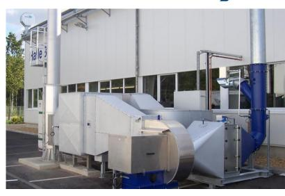
Catalytic incinerators are used to treat exhaust air, for example from the print, chemical and pharmaceutical industries as well as from various painting and coating systems.
