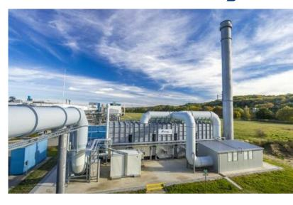
RTO units with two, three or more chambers are used in all industries that emit VOCs. They can be used for a wide concentration range and operate very economically, even without additional external heat recovery.
