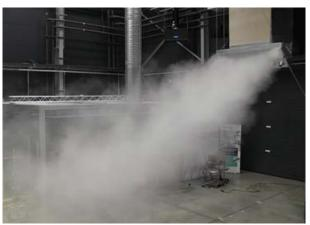
Figure 4: Setting for higher air movement in summer or for heating
