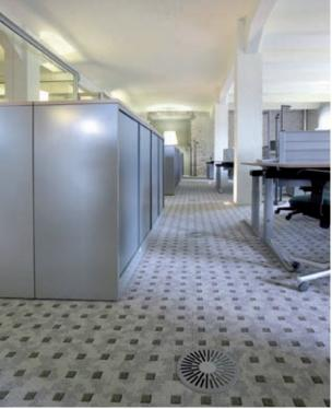
Figure 6: Floor twist outlet in an office
