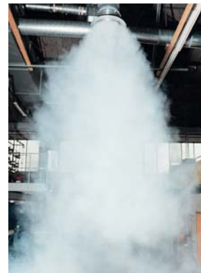
Air jet pattern of DD-VL below: horizontal discharge (cooling mode) left: vertical discharge (heating mode)
