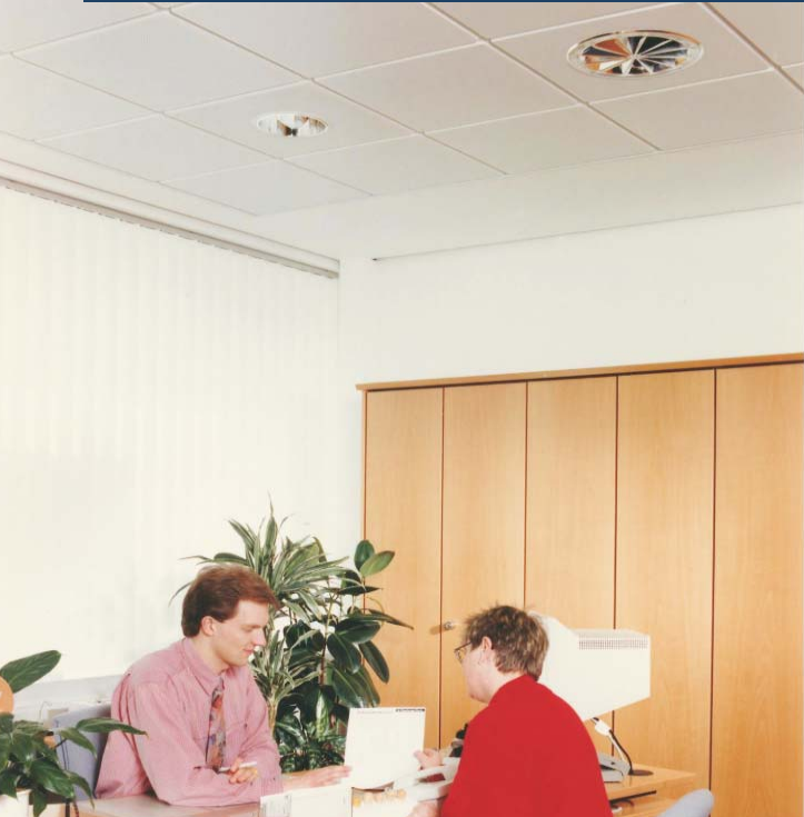
Radial outlet of type RA-N, chrome-plated, at the Hamburger Bank, branch office Osterstraße, Hamburg / D
