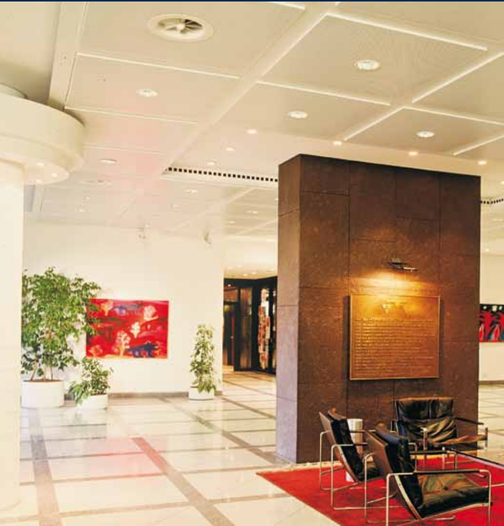
Ceiling air outlets Turbulent mixing air flow
