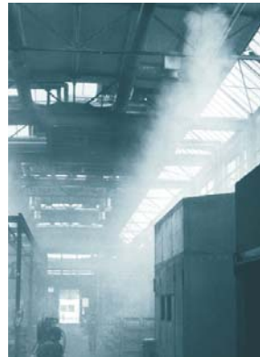
Air jet pattern of DD-VK below: horizontal discharge (cooling mode) left: vertical discharge (heating mode)
