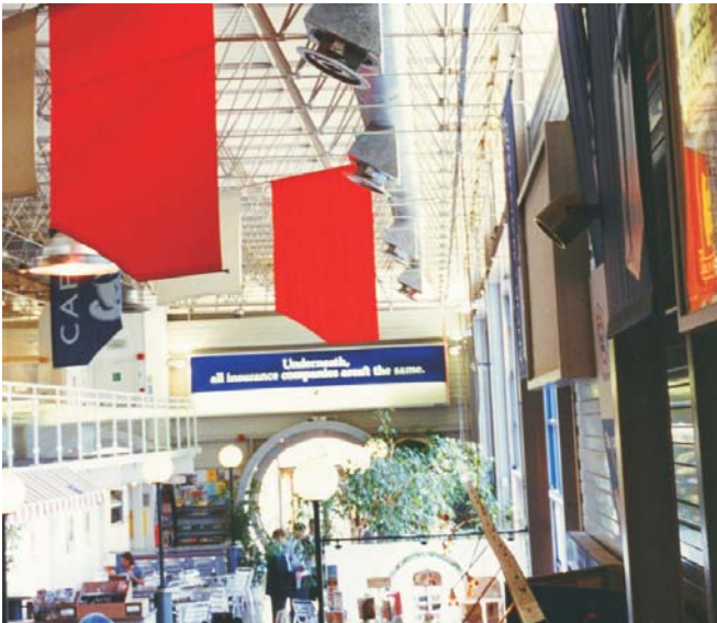
Variable twist outlet with core tube, type DD-VK, in the Channel Tunnel
