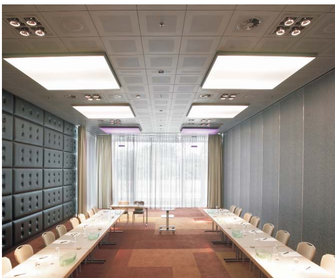
Adjustable radial outlet, type RA-V, at the Radisson SAS Hotel, Cologne / D
