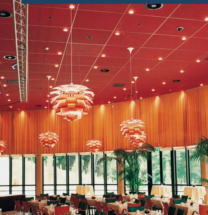
Adjustable radial outlet, type RA-V, in the restaurant at Holland Casino, Valkenburg / NL
