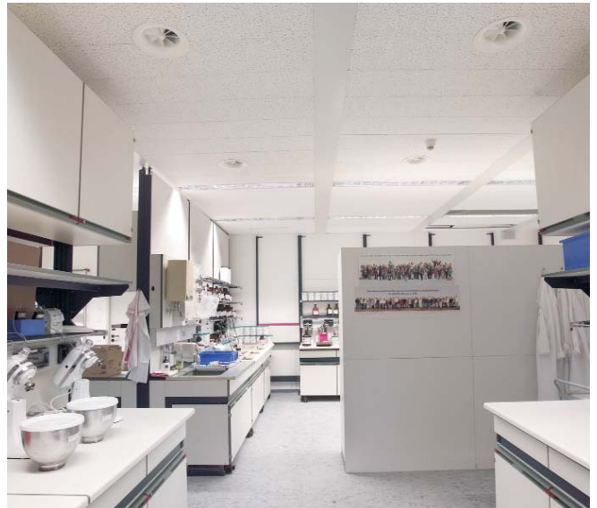
Twist outlet, type DD-N, at Beiersdorf AG, Hamburg / D
