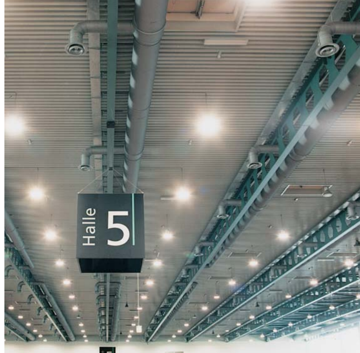
Variable twist outlet with guide ring, type DD-VL, in an exhibition hall of Bremen Fairgrounds / D
