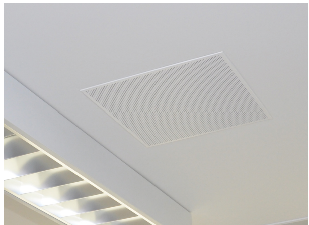
Fig. 7: Opticlean installed in a gypsum plasterboard ceiling
