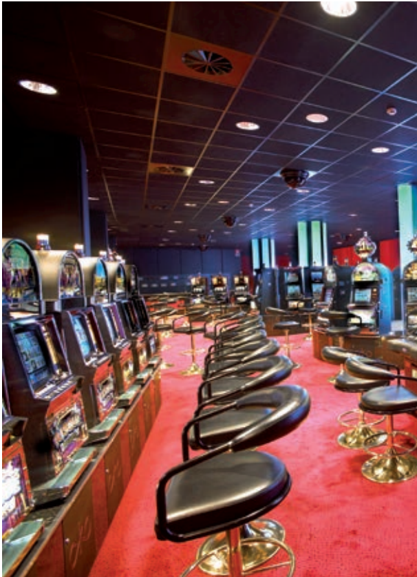
Radial outlet with square face in a casino
