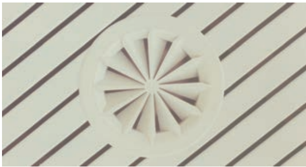
Radial outlet in a strip ceiling
