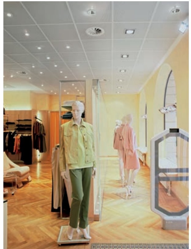
Radial outlet with circular face in a boutique
