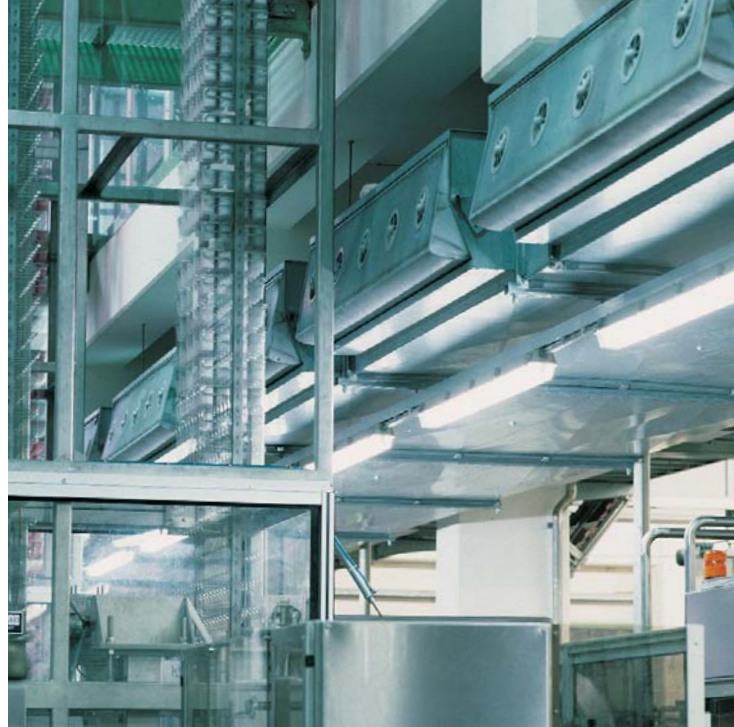
Swivel displacement outlet, type VA-S, in a production hall of the dairy 'Südmilch AG', Heilbronn / D
