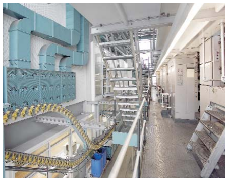
Rectangular displacement outlet, type VA-RN, in the printing shop of 'Vorarlberger Medienhaus', Schwarzach / A
