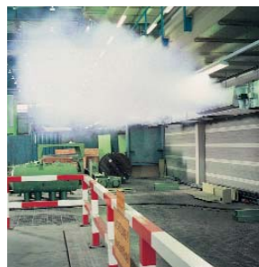
Air jet pattern of VA-S Cooling mode
