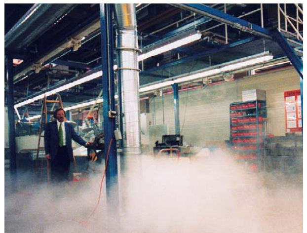
Circular displacement outlet, type VA-ZD, on the floor of the production hall of 'Stihl & Co.' at Wil / CH
