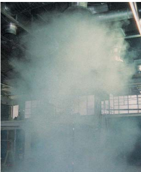
Air jet pattern of VA-PV Cooling mode
