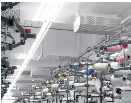
Trapezoidal displacement outlet, type VA-T, at 'Wolford AG', Bregenz / A
