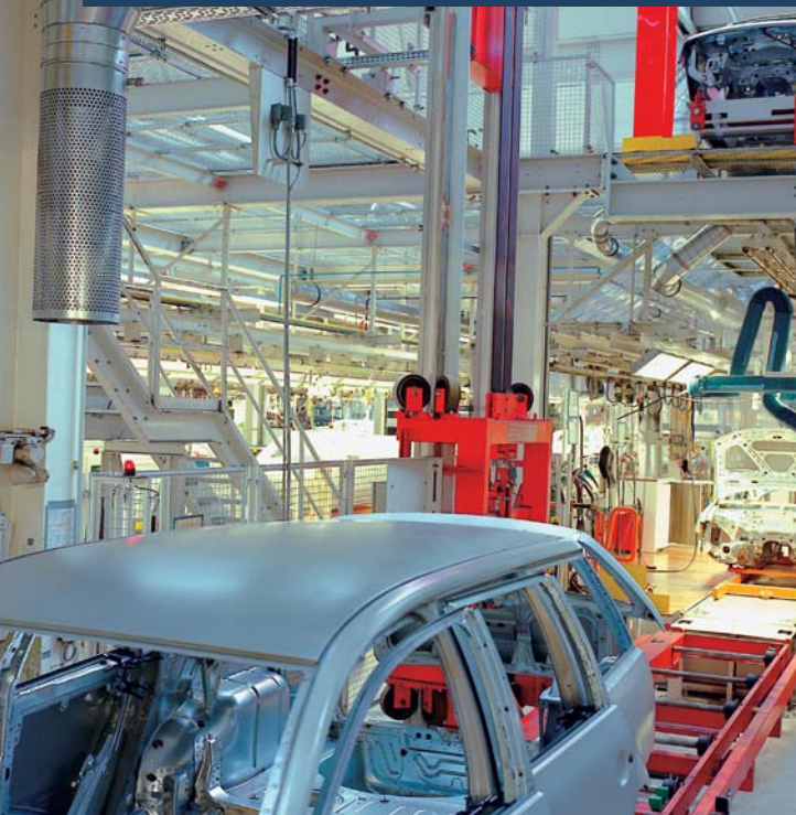
Circular displacement outlet, type VA-ZD, in a production hall of VW at Emden / D
