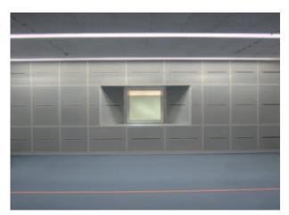
Air distribution wall with perforated discharge panels and linear slot diffusers
