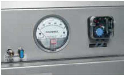
Magnehelic® differential pressure gauge for indication of filter loading
