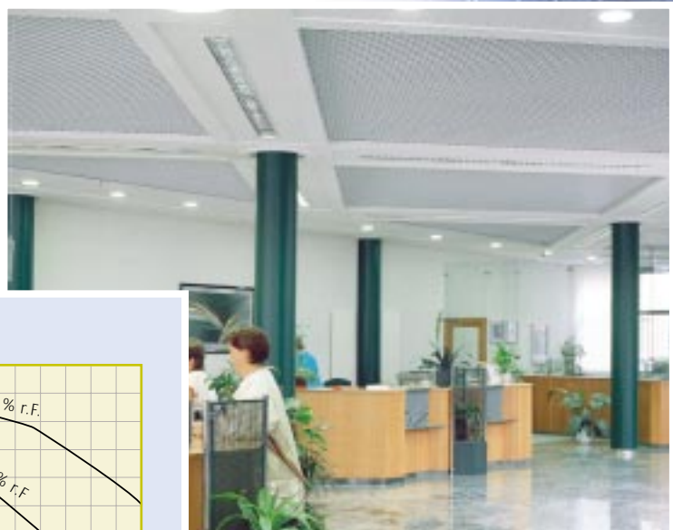
Grid ceiling with gypsum plasterboard frieze, combinable with SKS cooling elements
