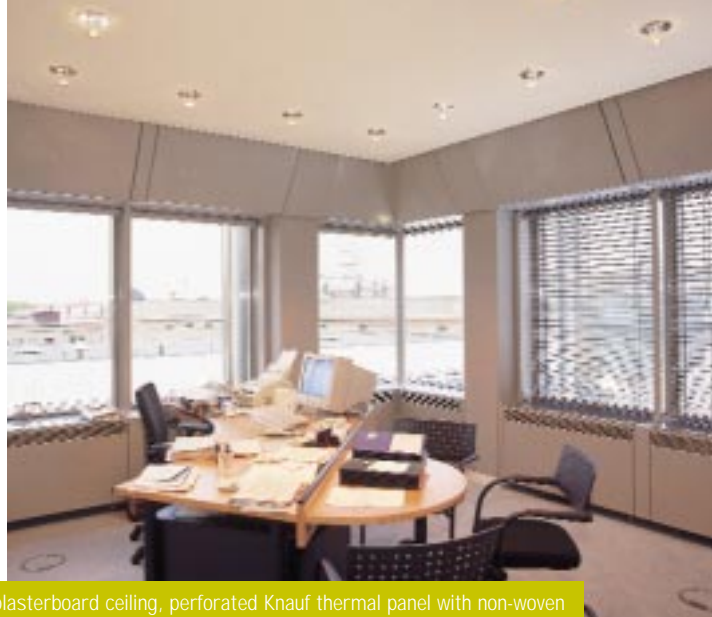
Gypsum plasterboard ceiling, perforated Knauf thermal panel with non-woven fabric and Scherf acoustic plaster, combinable with KKS cooling elements
