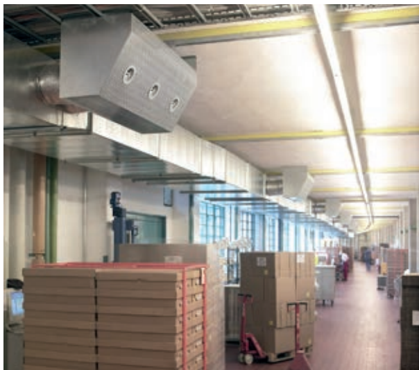
Figure 12: Semi-trapezoidal displacement outlet of size 500 in a production facility
