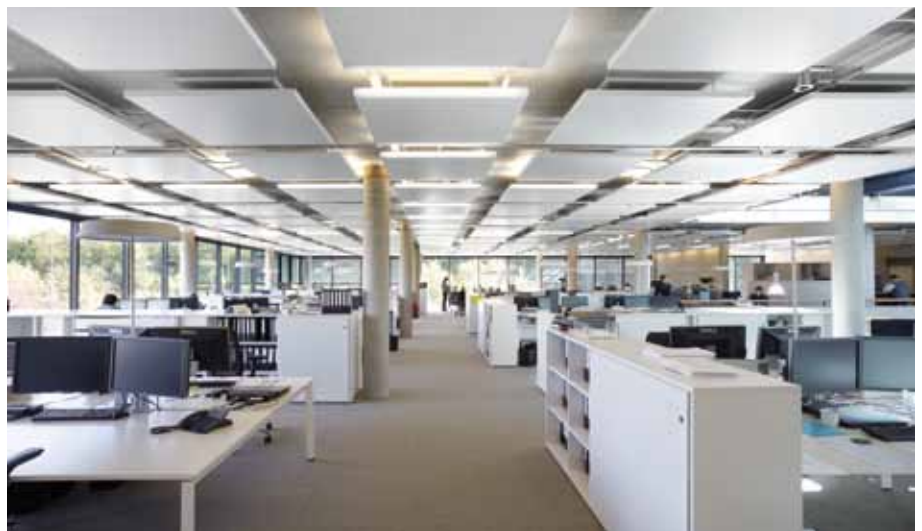
Multifunction exposed ceiling
