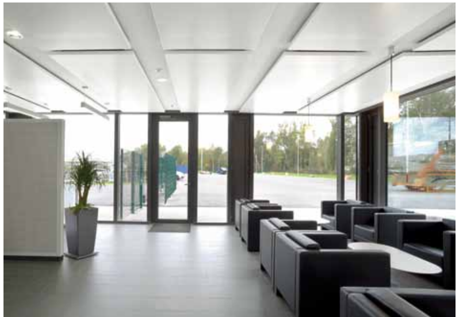
Multifunction exposed ceiling
