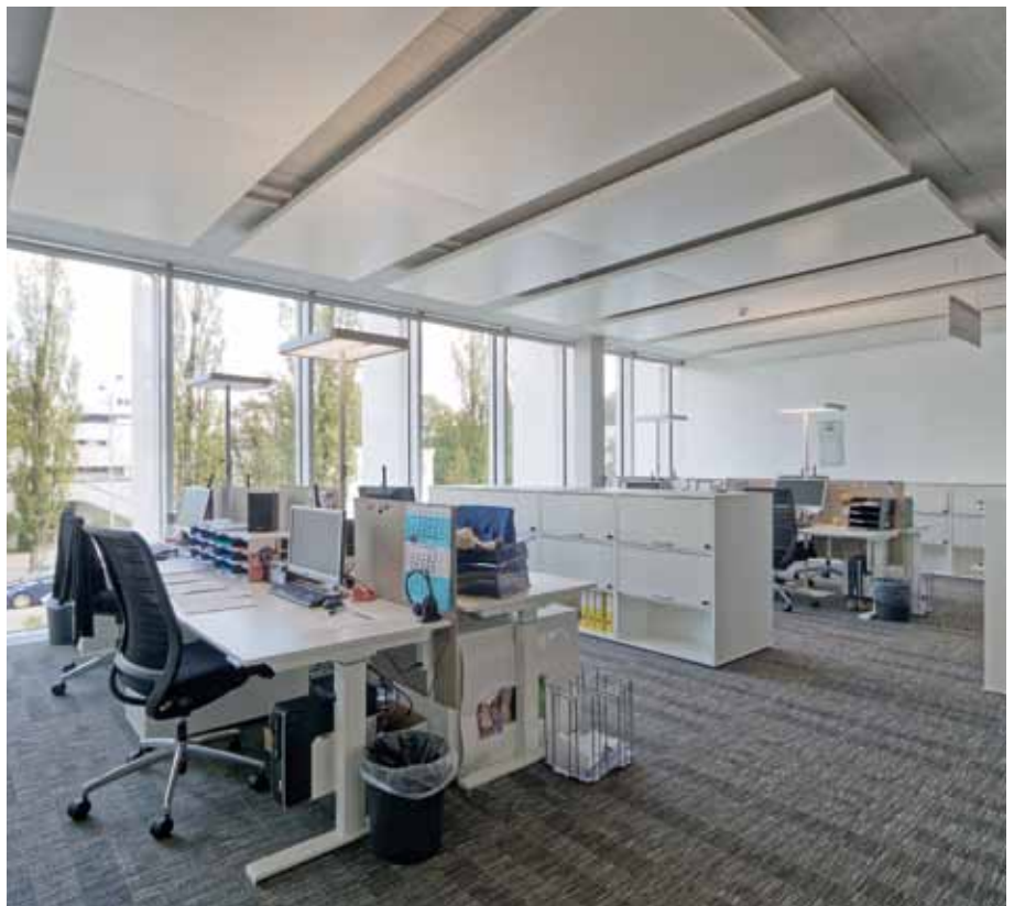
Multifunction exposed ceiling
