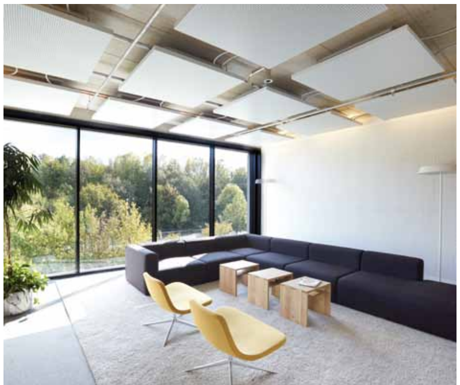
Multifunction exposed ceiling
