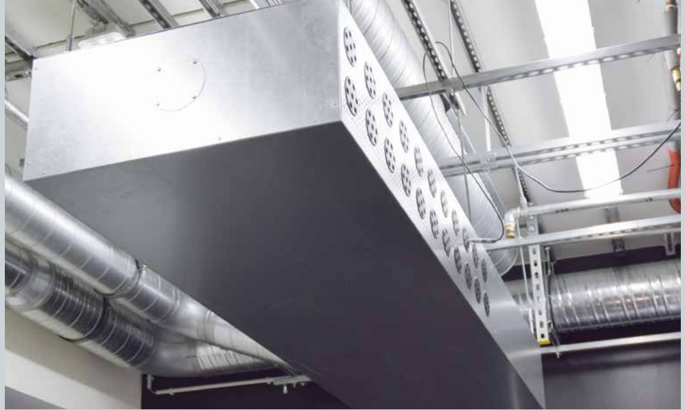
Laboratory outlet with two-row configuration
