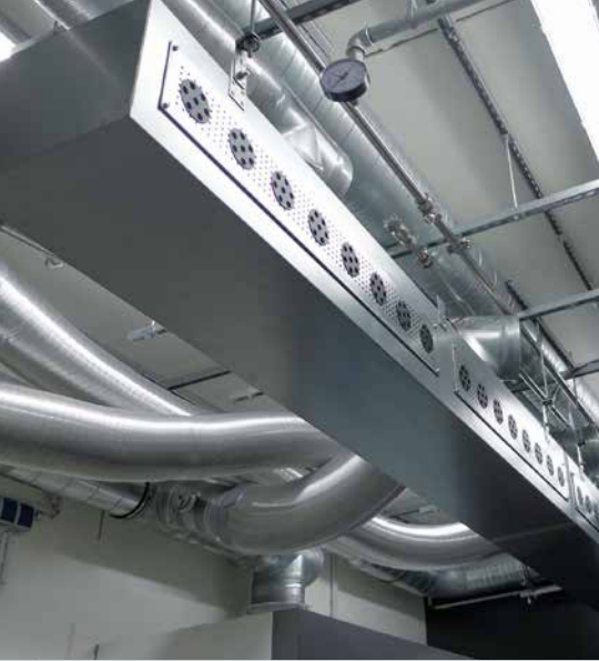
Laboratory outlet with single-row configuration
