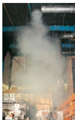
Air jet pattern, vertical discharge (heating mode)
