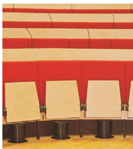
Seat displacement outlets at the 'Konrad-Adenauer-Stiftung', Berlin / D
