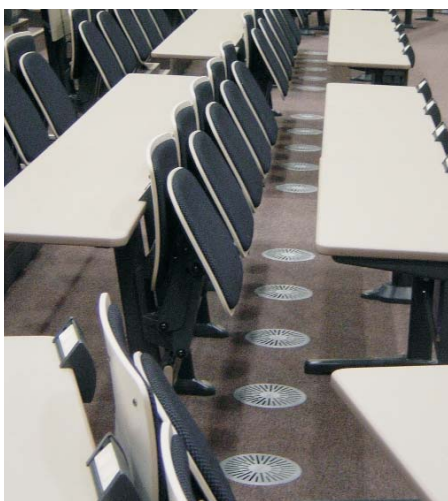
Floor twist outlets at the University of Osaka / J
