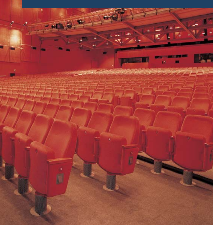
Seat displacement outlet, type Q-St, in the 'Stella Musical Theater', Berlin / D
