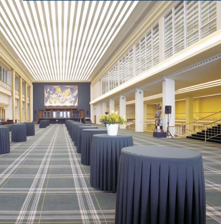
Linear whirl outlets in the Hall of Honour of 'Casino Kursaal Ostende' / B
