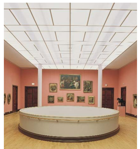
Plinth displacement outlets at 'Kunsthalle Bremen' / D
