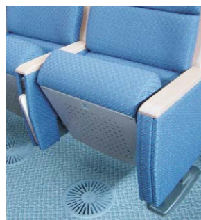
Floor twist outlet, type DB-E, in the media centre of Osaka University of Commerce, Osaka / J
