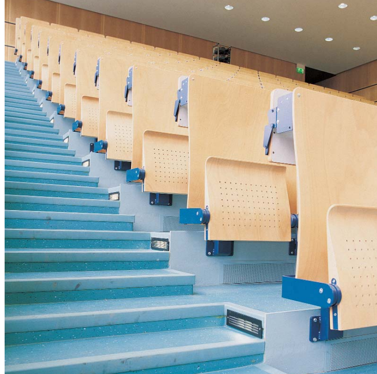
Step displacement outlet, type Q-SL, in a lecture hall at the Lausitz University of Applied Sciences, Cottbus / D
