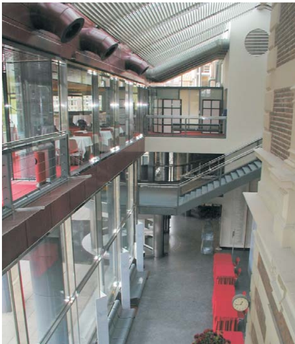
Twist outlets in the foyer of 'Het Concertgebouw', Amsterdam / NL
