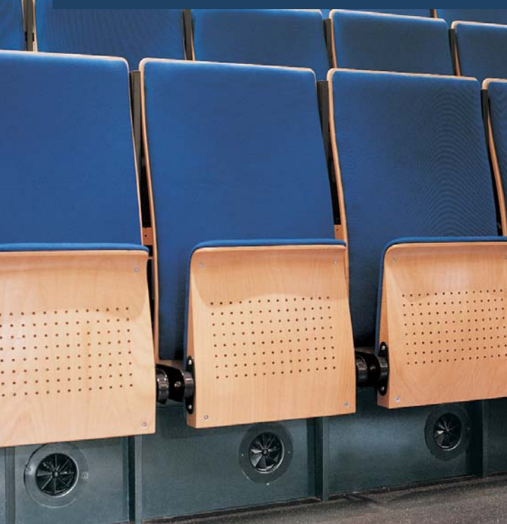
Step twist outlet, type DS-DD, in a lecture hall at the University of Amsterdam / NL
