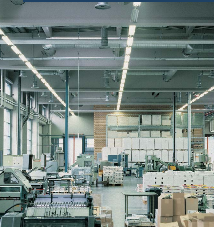
Radial displacement outlet, type VA-PV, in the printing shop of 'Frankfurter Societät', Mörfelden / D
