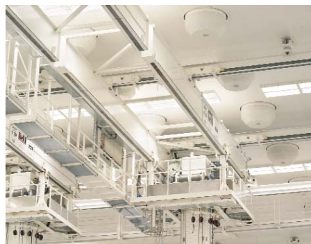
Conical displacement outlet, type VA-K, in an aircraft painting hangar of 'Deutsche Airbus', Hamburg / D
