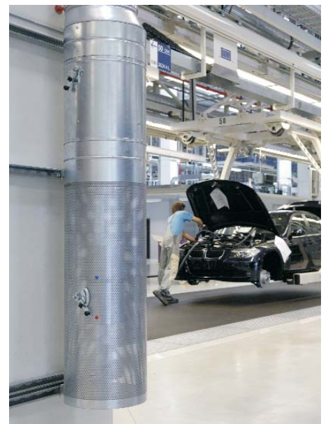
Circular displacement outlet, type VA-ZD, at 'BMW AG', Leipzig / D (Photographer: Martin Klindtworth)
