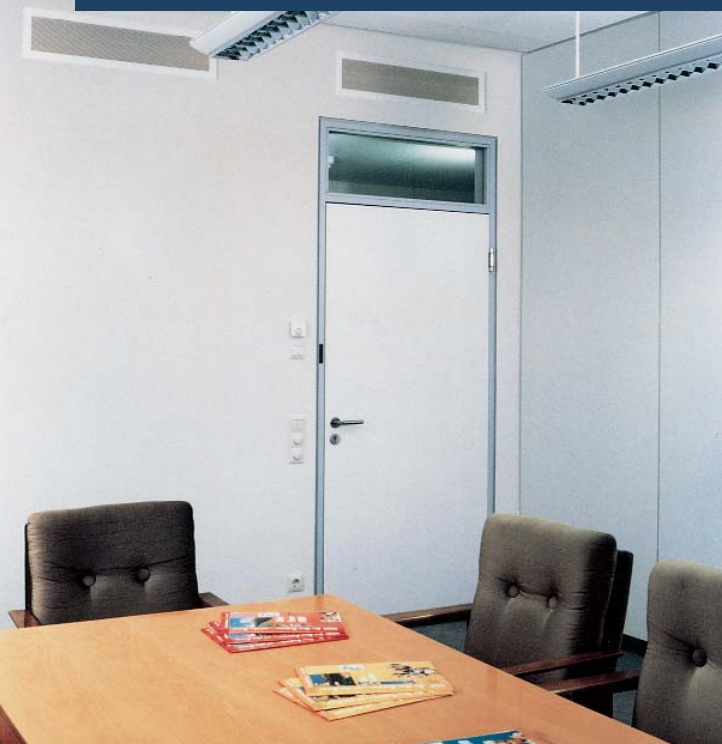
Wall displacement outlet, type Q-WL, in a meeting room
