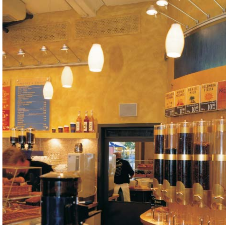
Multiplex displacement outlet, type FA-VQ, in a Tchibo coffee shop in Berlin / D
