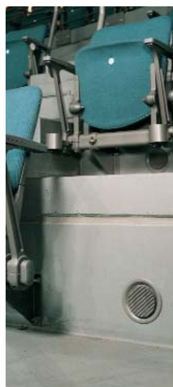
Step displacement outlet, type Q-SR, at 'Kölnarena', Cologne / D
