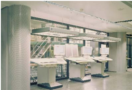
Semi-circular displacement outlet, type Q-ZH, in the restaurant of the business park at Mägenwil / CH
