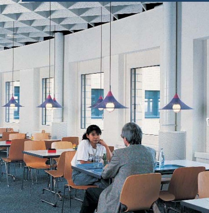
Semi-circular displacement outlet, type Q-ZH, in the restaurant of the business park at Mägenwil / CH
