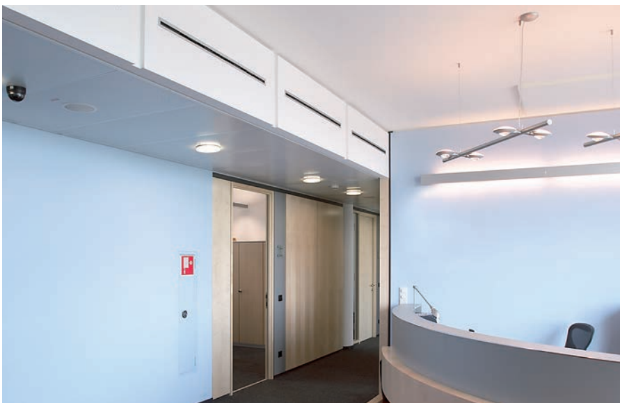
Wall slot diffuser WSD
