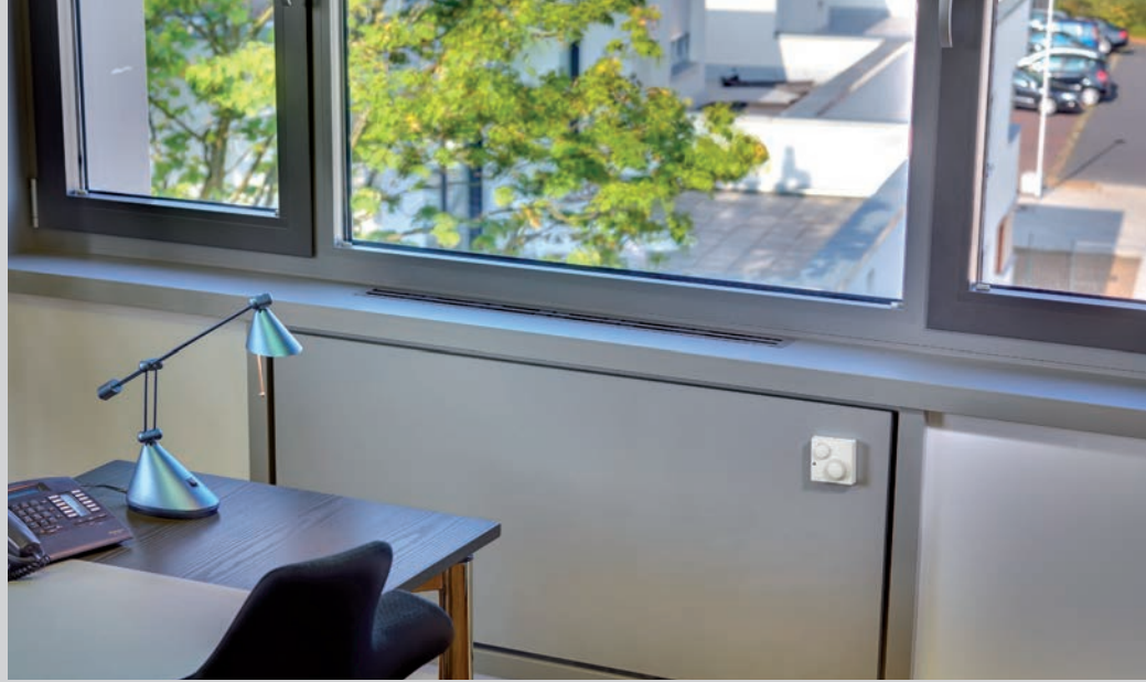
Ventilation unit (supply/return air) for mixing ventilation LG-ZA-M-SB, for vertical parapet mounting
