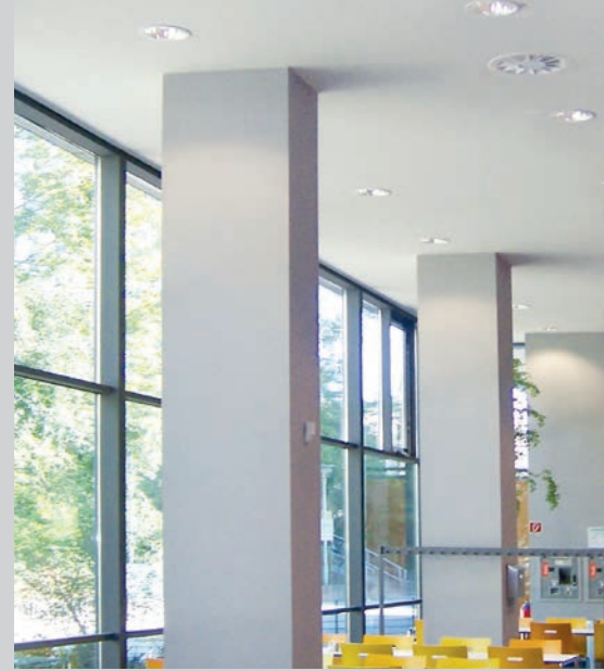
Adjustable radial outlet with core tube RA-V2
