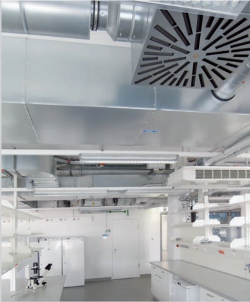
Radial slot outlet RL
